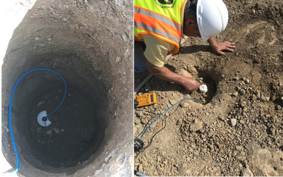
Figure 16. Instrumentation of the geophones in the subgrade.
